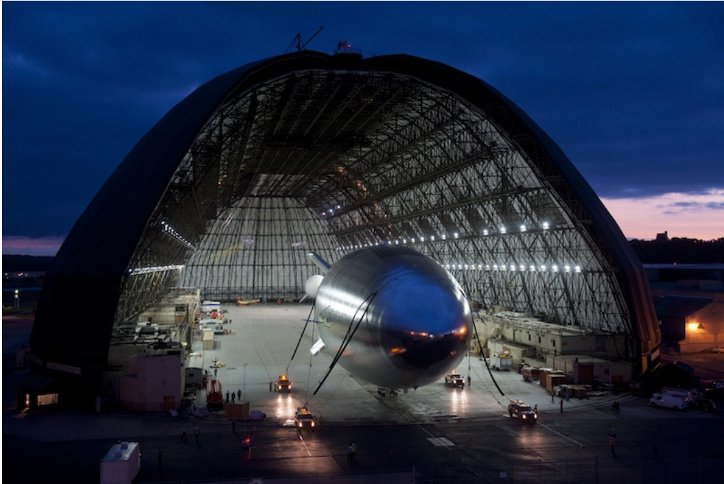
Figure 6-1 - Airship Hangar build in 1929 in Akron, OH refurbished by Lockheed Martin in 2011
